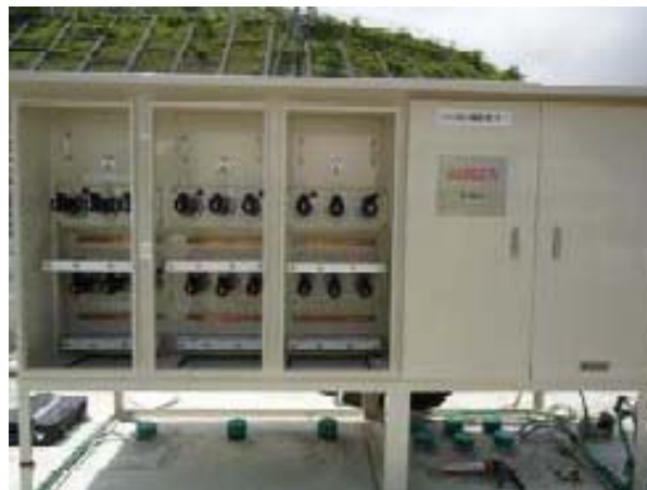
Power supply inlets outside of the buildings (Source: The Shikoku Electric Power Co.,Inc.)
