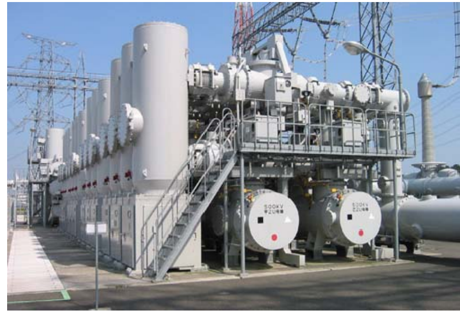
550kV gas insulated switchgear (GIS)
