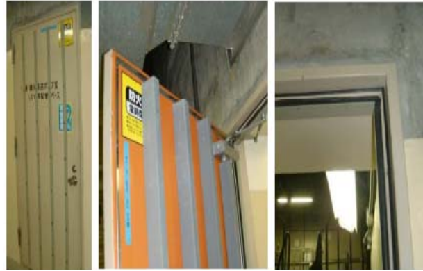
Watertight door (Source: The Chugoku Electric Power Co.,Inc.)
