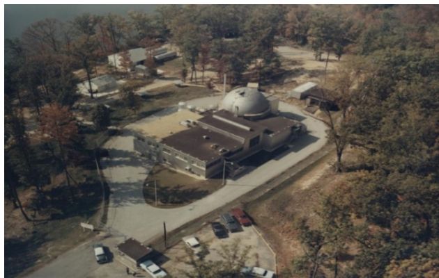
A view of the SM-1 reactor on Fort Belvoir
